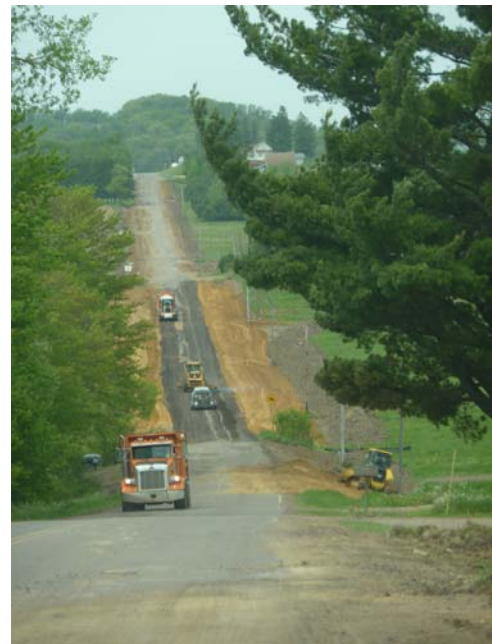
County Highway B Reconstruction May 2012
